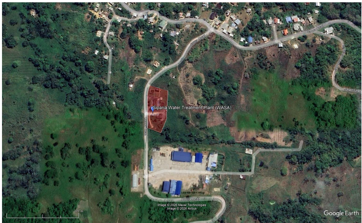
Figure 4-25: The Siparia Water Treatment Plant and surrounding environment
