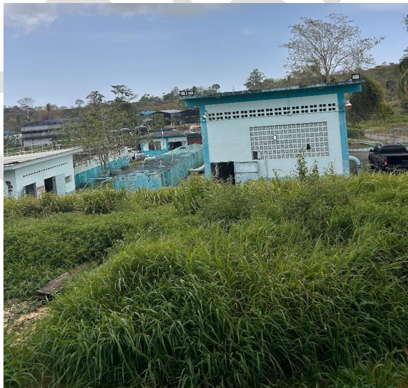
Figure 4-26: Vegetation on sections of the Siparia Water Treatment Plant
