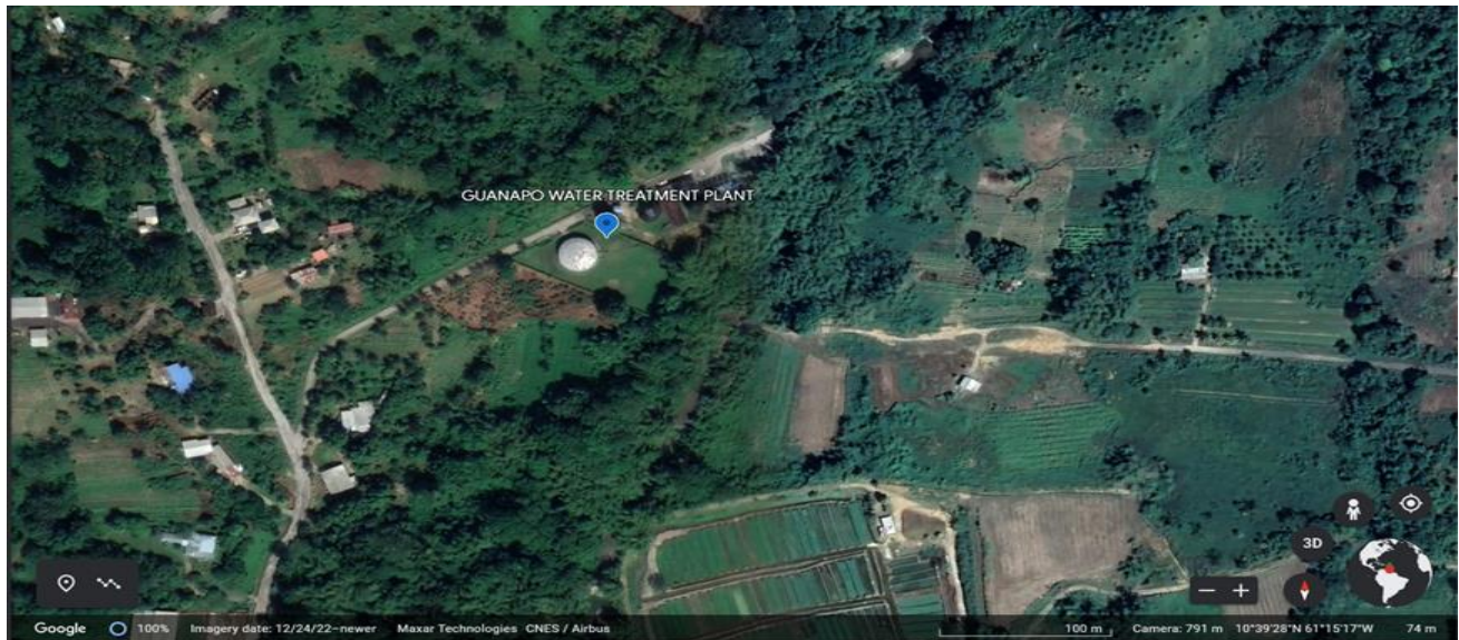
Figure 1: Site of the Guanapo Water Treatment Plant
